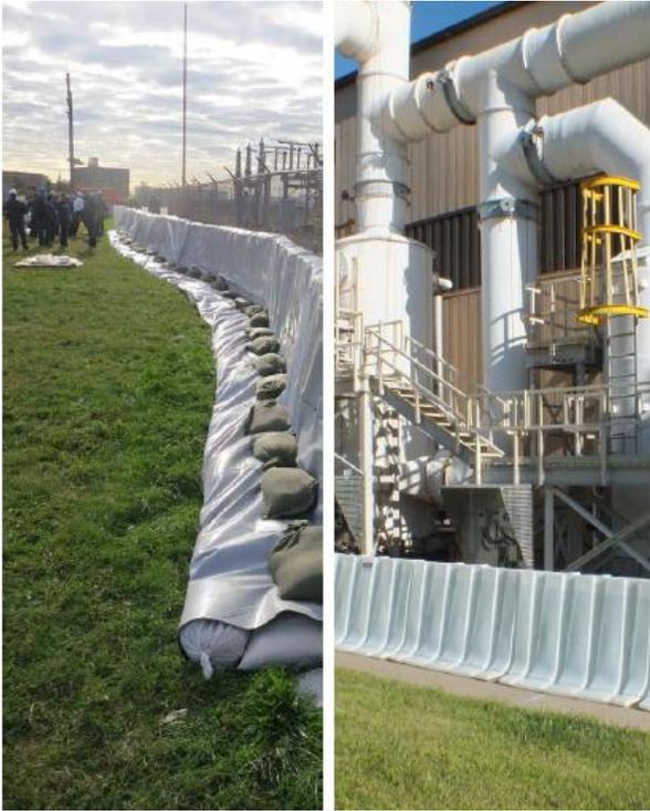
Figure 8. The temporary "muscle wall" erected to protect the PVSC treatment plant in July of 2013 would be replaced with a permanent flood wall as part of the PVSC's Flood Mitigation Plan. (Source: "Recovering from Superstorm Sandy," PVSC, January, 201
